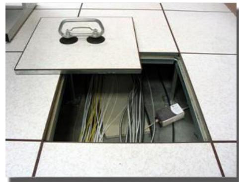
Figure 8. Connection of ground line filters
